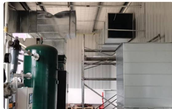
Pipe connecting the heat outlet of the air compressor with the molding room
