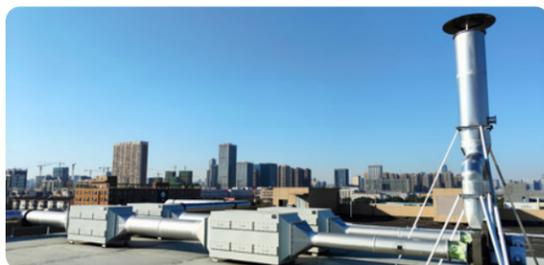
Grade 2 activated carbon adsorption + exhaust funnel P203
