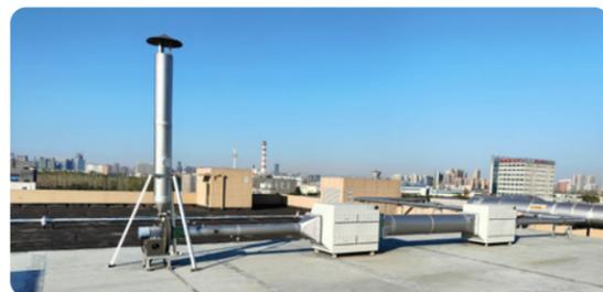
Grade 2 activated carbon adsorption + exhaust funnel P204
